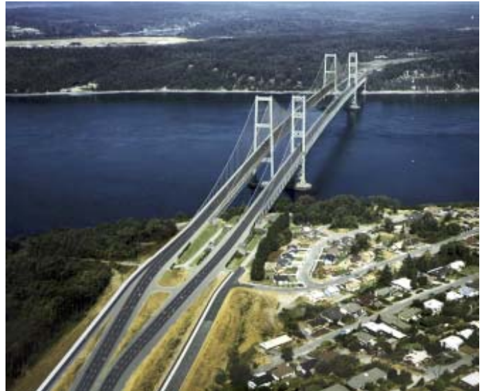
SR 16 - New Tacoma Narrows Bridge, Washington
